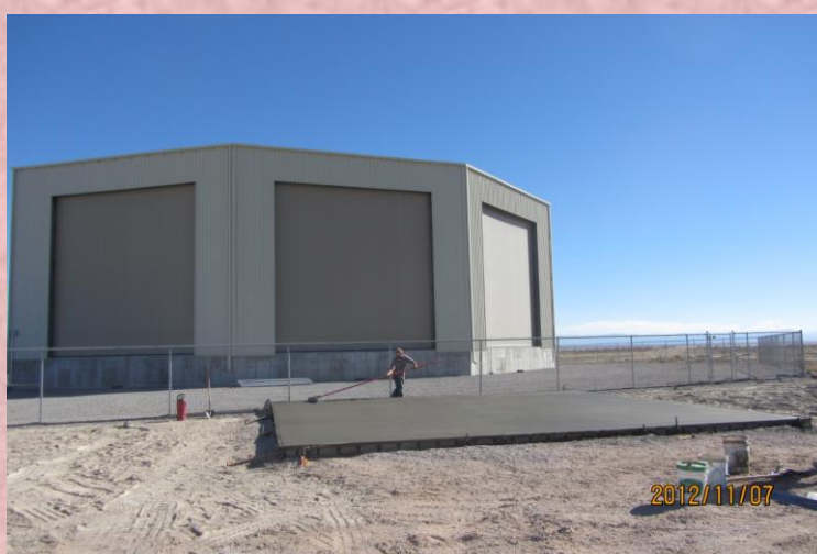
The concrete pad is prepared by TA group.
