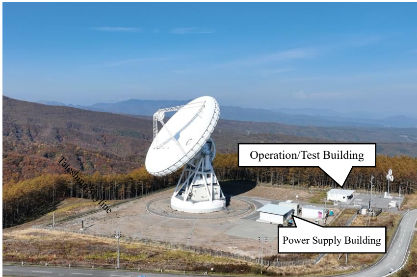
Figure 3-1 MDSS (From North)
