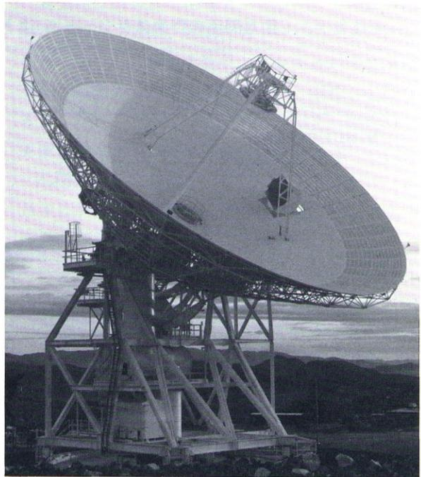
Fig. 3 The New 34-m Research and Development Antenna
